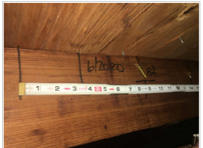
8d Nails within 6"
